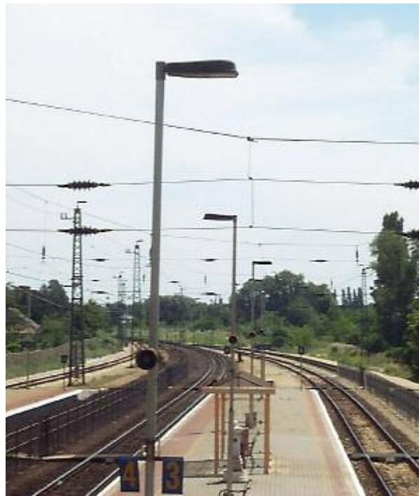
Figure 1. The new luminaires at a railway station. Note the very flat structure of the light fixtures. Courtesy TUNGSRAM-Schréder.
